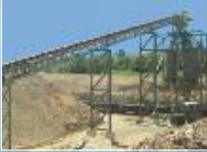
RAILCAR LOADING SYSTEM
