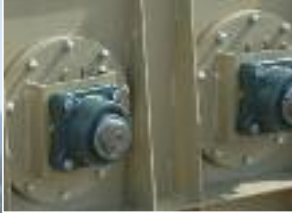
STIFFENERS STRENGTHEN TANK
